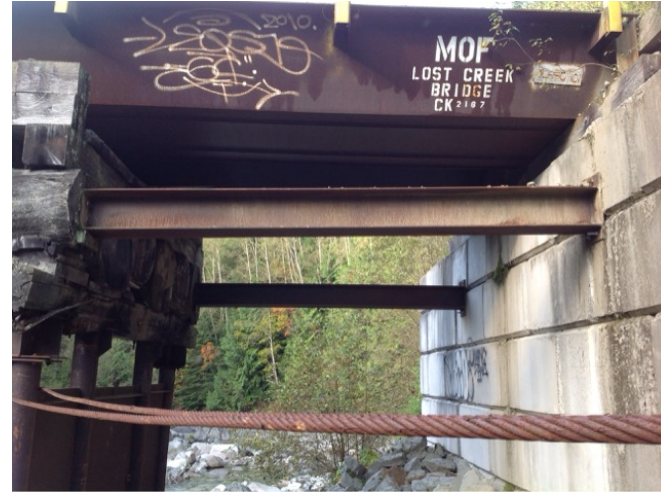
old log stringers fastened to lock block abutments
