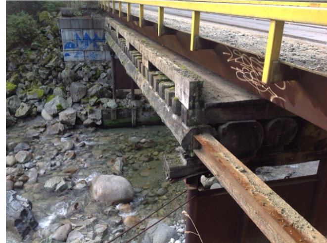
old structure underneath
