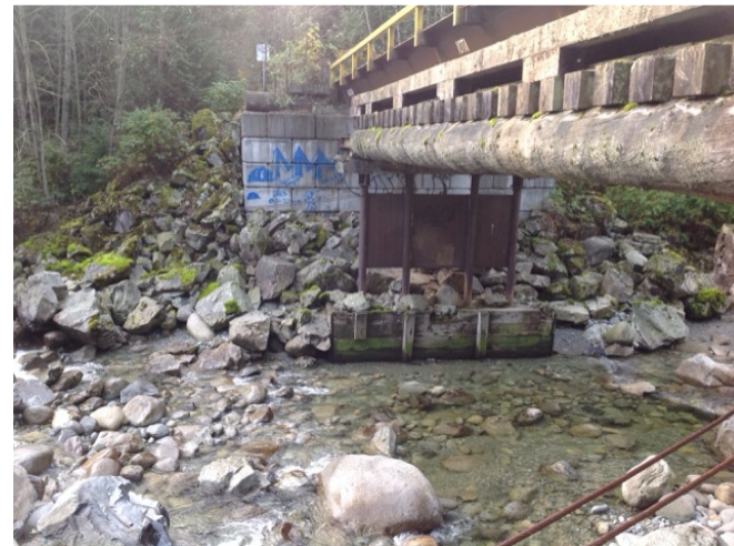
Left Bank Abutment when facing downstream
