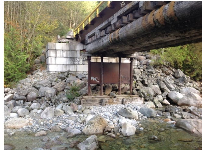
Right Bank Abutment when facing downstream
